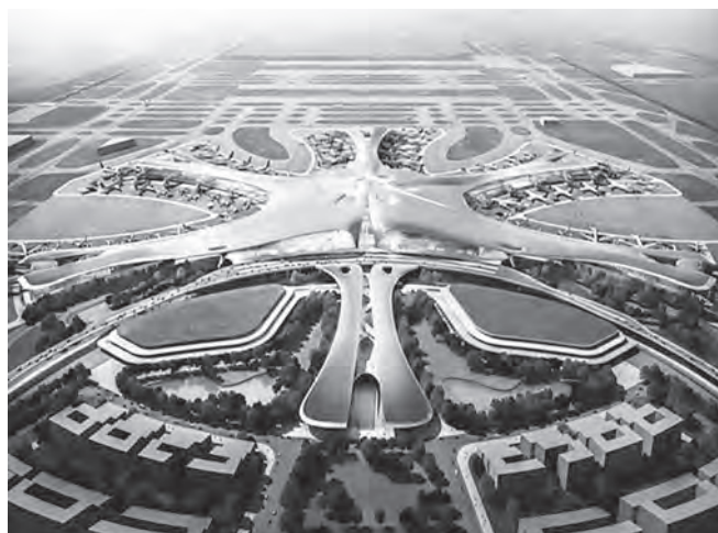
The new airport in Beijing-Daxing should open in 2019.
