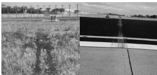
Contact marks on overrun area and runway.
